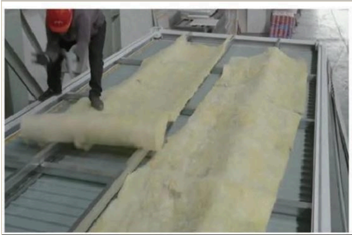
FIG. 5.2 Fibreglass foil insulation rolled on top of the plastic sheet.
