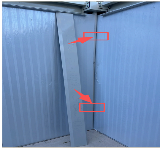
FIG. 9.1 Column cover panel (CH-COL-018) being fitted over the corner metal angle — arrows highlight the snap-fit edges that must engage along the column length.
