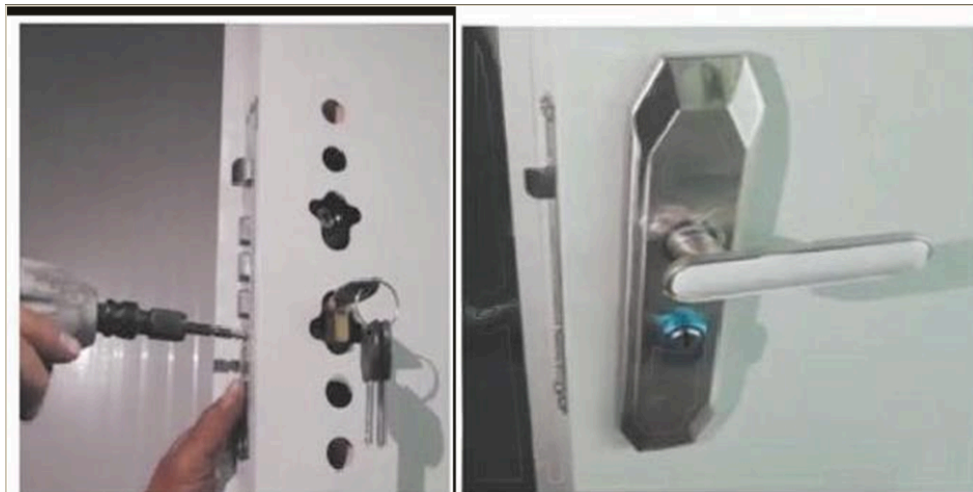
FIG. 9.2 Door lock installation — secure the lock body with screws (left), then fit the handle and cylinder (right) and test before sealing.
